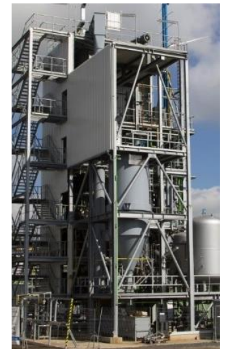
FlexiSlag Pilot Plant © IEC
