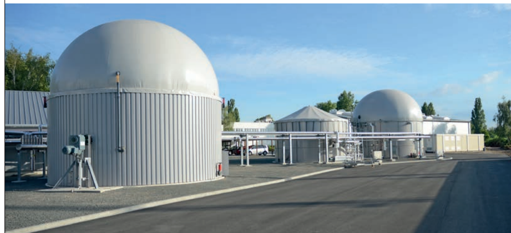
Fig. 6 DBFZ research biogas plant (continuous stirred tank reactor with pneumatically supported double membrane gas storage roof at front left)
