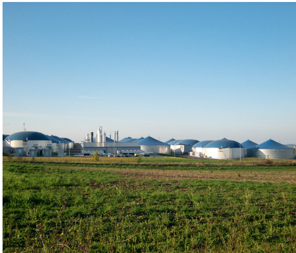
Fig. 31 Biogas treatment plant with biomethane supply
