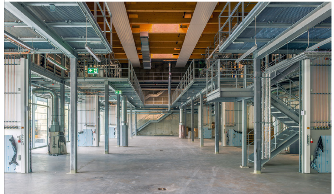
Fig. 42 New conference centre and pilot plant hall (thermo-chemical conversion segment)
