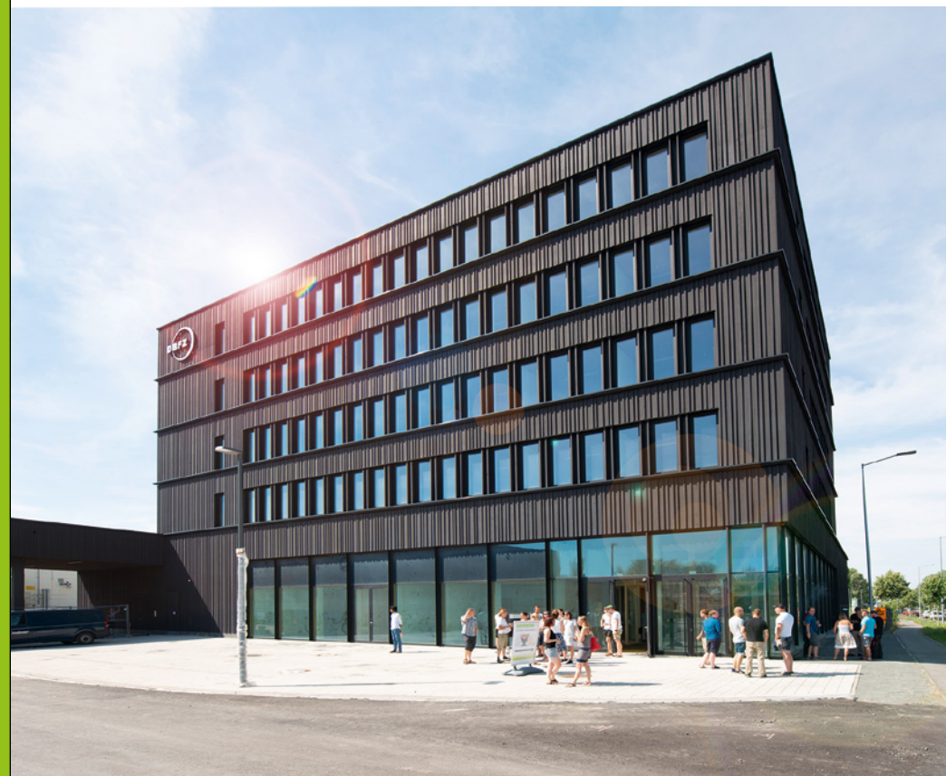
Fig. 41 The new building (House 1) of the DBFZ in March 2019
