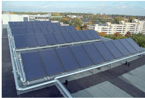
Solarthermie-Anlage © BSW
