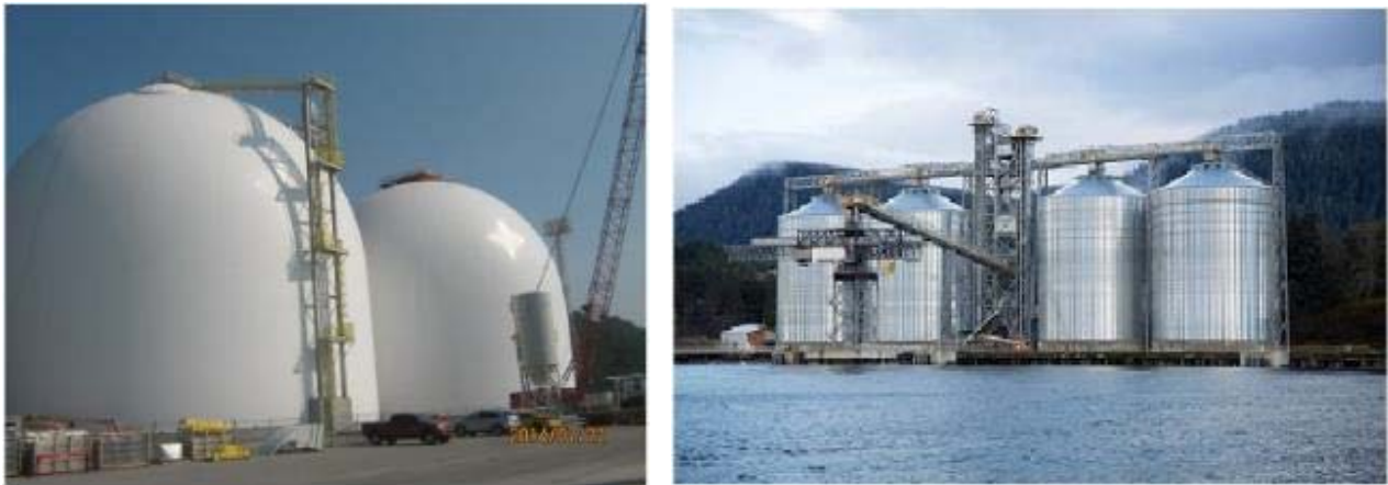
Figure 7 Left side; Quebec Stevedores, Quebec City, 75 kt. Right side; Westview Pellet Terminal, Prince Rupert BC, 60kt
